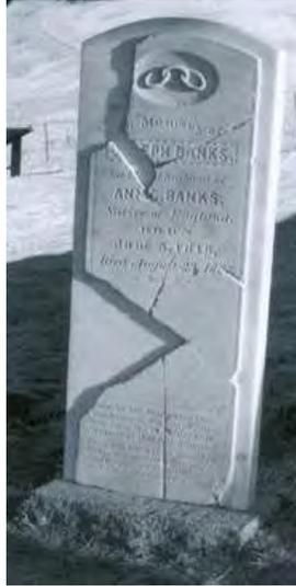
*The Joseph Banks stone repaired by the encasement method*
